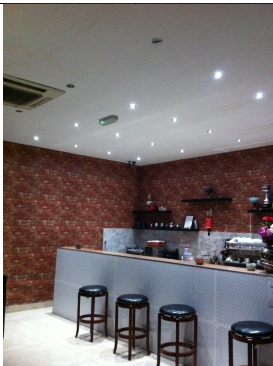
26 CCTV in the front corner of shisha smoking room
