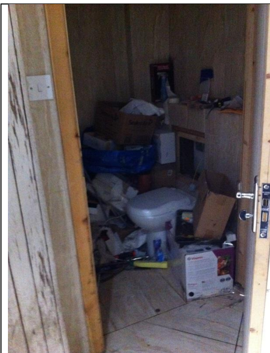
11 Disabled toilet – filled with rubbish
